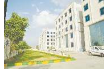
Apex South Campus - III IS-2018, Ramchandrapura, Sitapura Ext., Jaipur-303905
